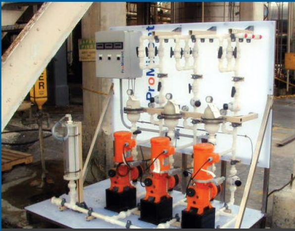
Metering systems for a chemical additive
