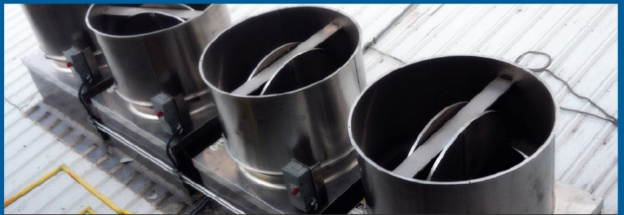
Direct drive stainless steel exhausters on asphalt fumes
